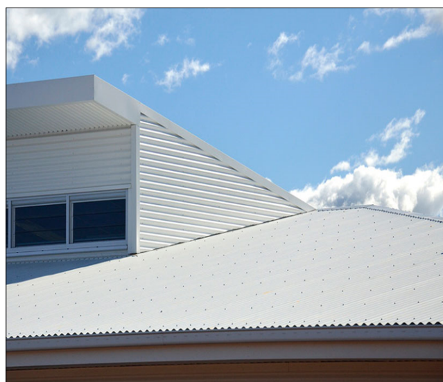
Figure 12 - Illustration of a light coloured (reflective) roof sheeting.
